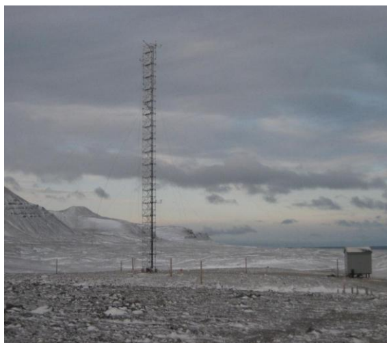
Photo 1: The Amundsen-Nobile Tower and the hut hosting computers and communication system.
